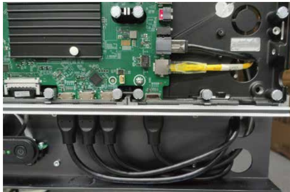
Suggested wire management plan for the terminals inside the lower rear front shell.
